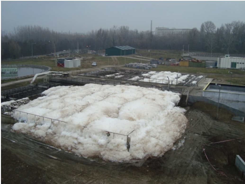
The reactor in the background contains the Organica Biomodules, where the one in the foreground is operated with activated sludge.
