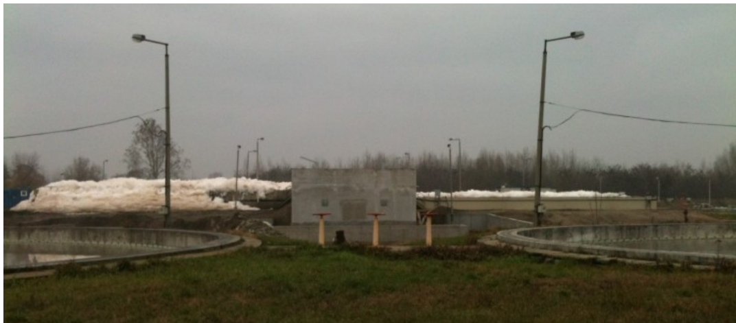
The reactor on the right contains the Organica Biomodules, while the one on the left is using activated sludge.
